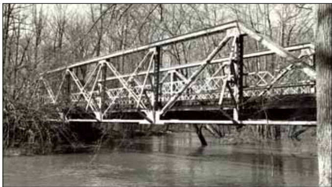
Duwall Bridge associated with the Duwall Mill (PG: 64-2).
